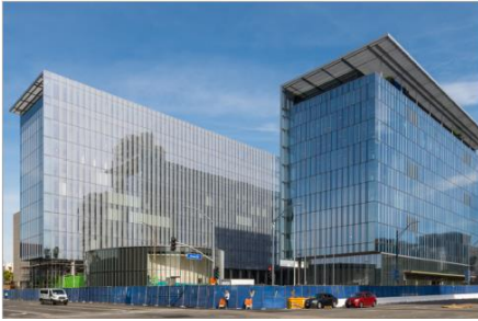
Long Beach Civic Center - Provided stair and associated rail design for the City Hall Building and the Library Building. Steel Fabrication Support, Construction Engineering
