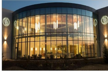
University of Delaware Star Labs - Provided the seismic analysis and equipment anchorage for a large, multi-story modular master plant located on the roof of the serviced structure. Existing Building Analysis
