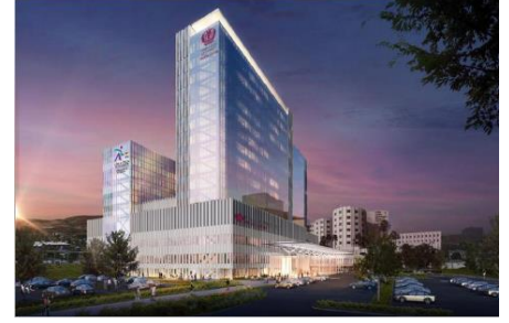
Loma Linda University Medical Center - Provided stair portion of the vertical circulation package for the new addition. Steel Fabrication Support, Construction Engineering
