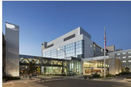
White Plains Hospital - Provided a mechanical enclosure on the rooftop that incorporates modular construction and supports davits, chillers, and other equipment. Structural Design, Existing Building Analysis
