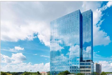
Fairmont Austin - Developed structural steel connections and vertical bracing. Steel Fabrication Support, Construction Engineering
